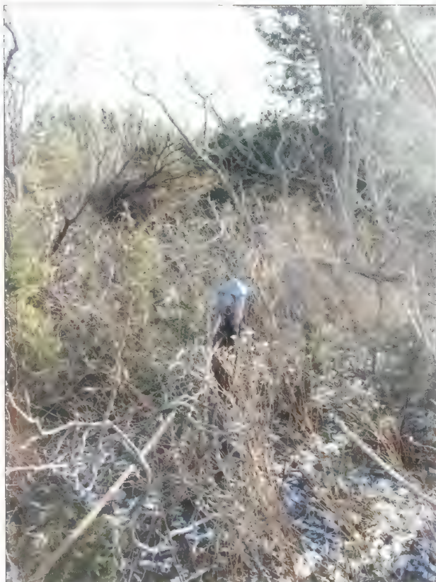
Figure 3.56. Post and wire fence, Battery Kingman. Near the high point above Battery Kingman's emplacement #2, a post and wire fence is installed that is overrun by vines and other vegetation (Olmsted Center, January 2009).
